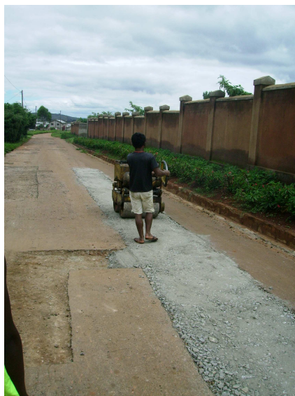
PHOTOS 72- Compactage GCNT 0/31.5
