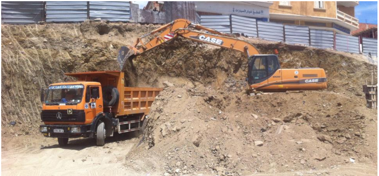
Figure 28: Excavation en masse.
